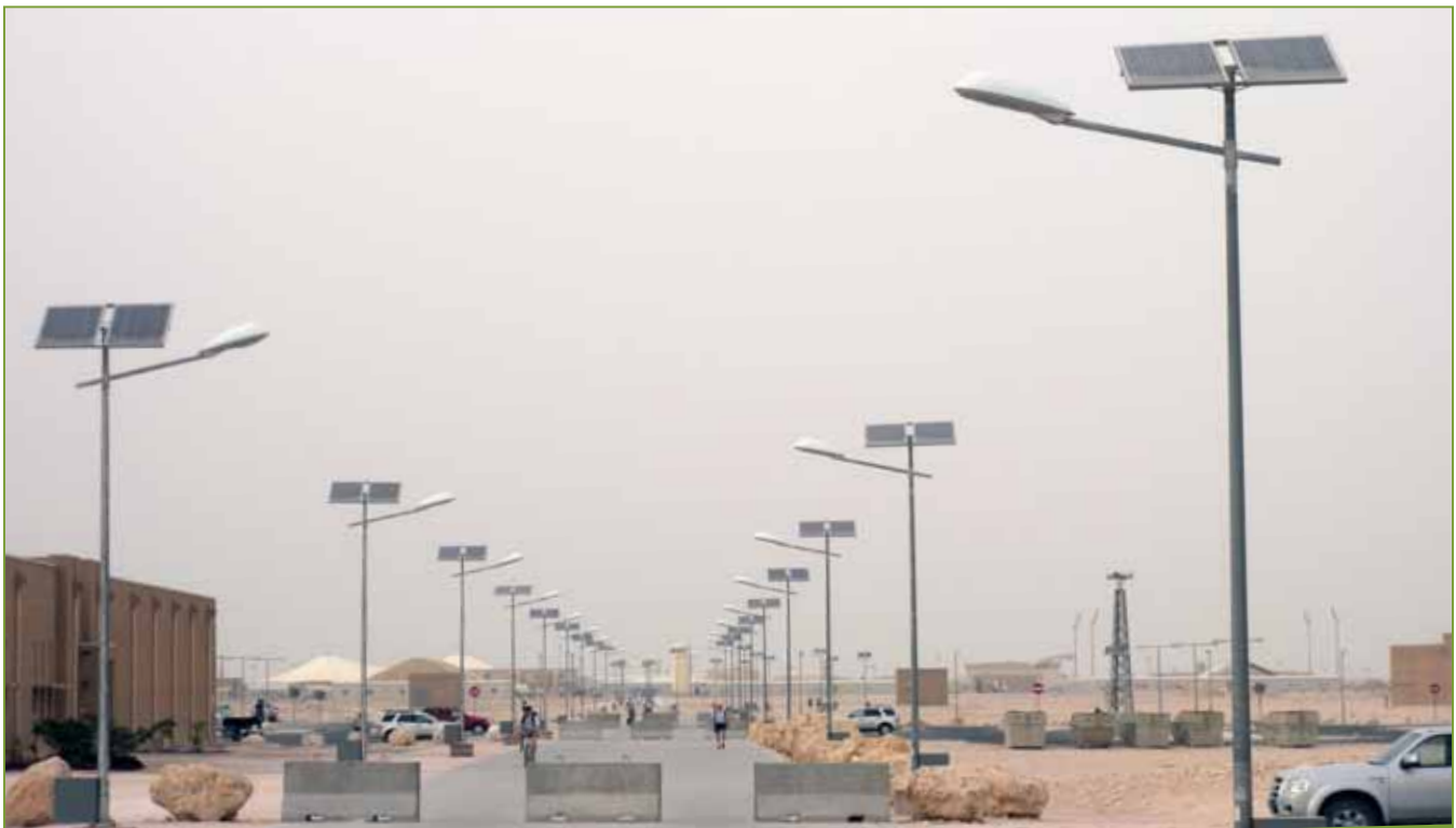
Solar lighting at Area Support Group-Qatar (photo: COL Anthony Haager).
